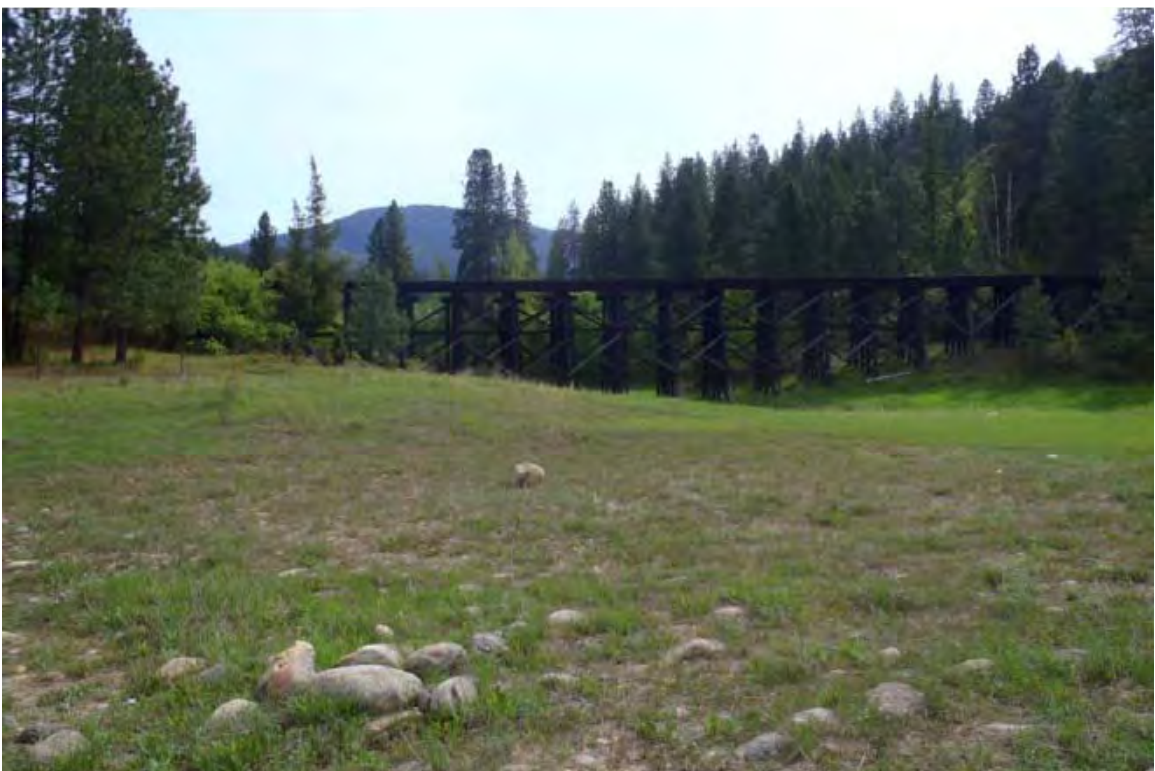
CH2M HILL Photo#98 - Onion Creek train bridge (P5080577)
