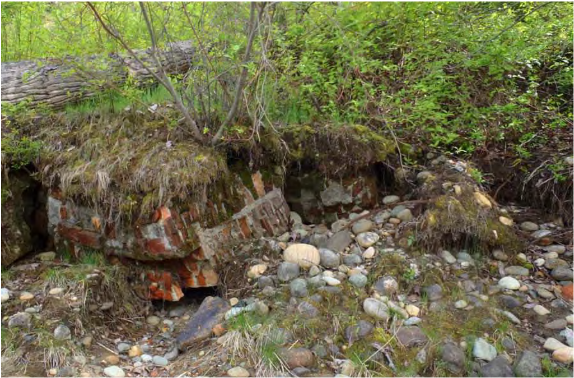
CH2M HILL Photo#93 - Northport - brick pipe work (P5080572)
