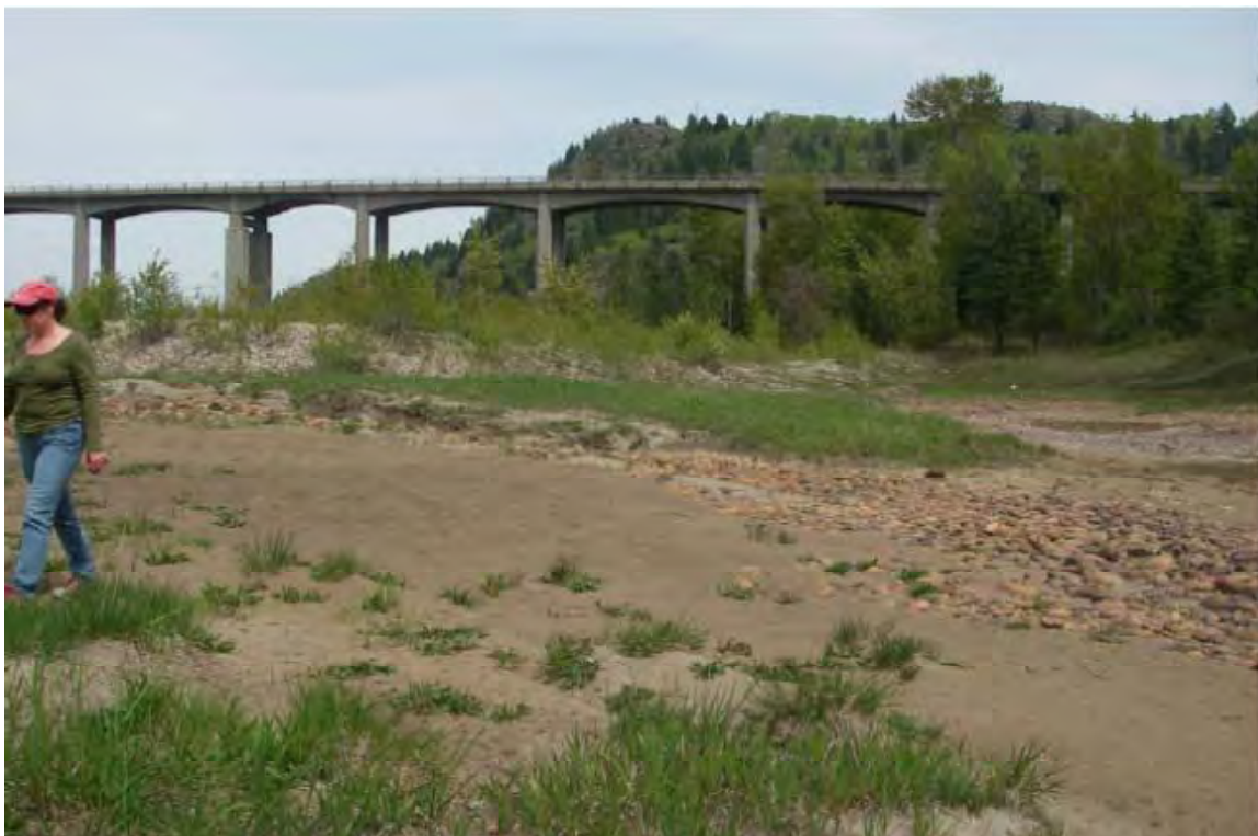
EPA Photo #61 - Marilyn - deposition/sand d/s of bridge (IMGP0061)
