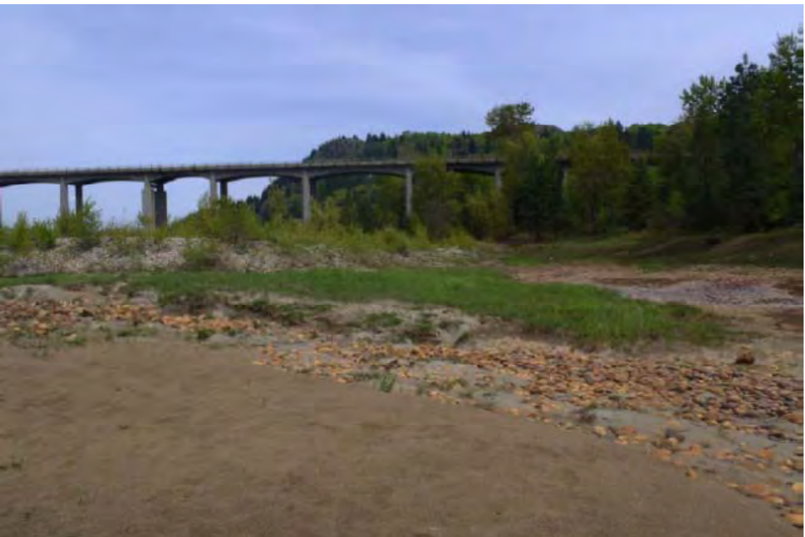
CH2M HILL Photo#84 - Northport - deposition/sand d/s of bridge (P5080563)
