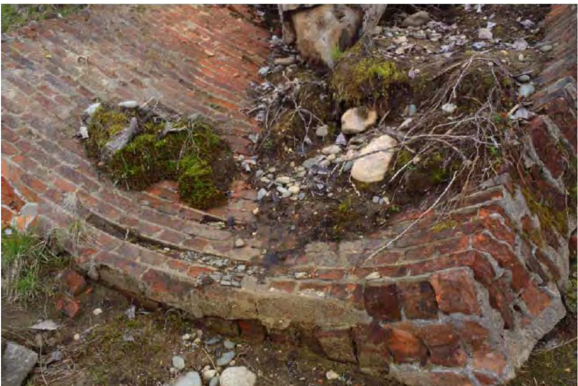
CH2M HILL Photo#94 - Northport - brick pipe work (P5080573)
