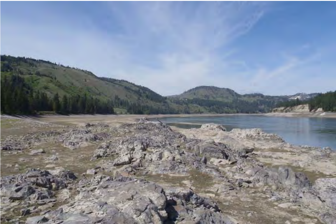
CH2M HILL Photo#25 - from bedrock south of Snag Cove (P5070504)
