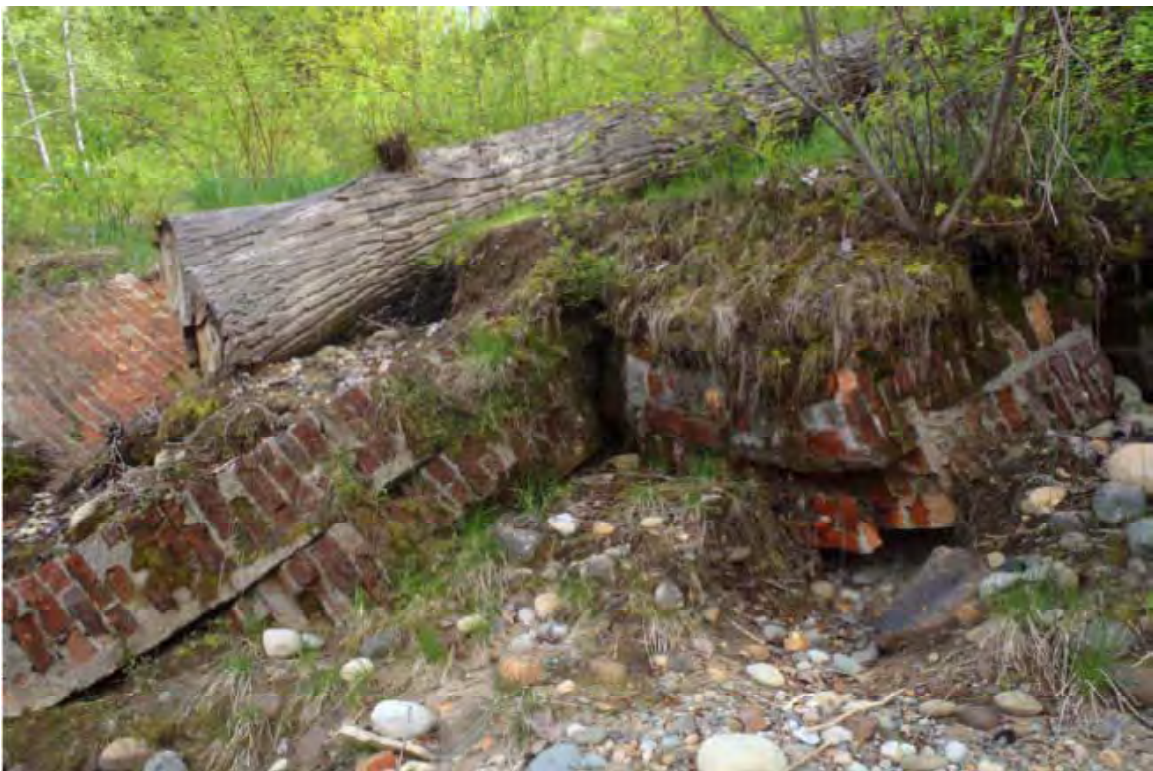
CH2M HILL Photo#92 - Northport - brick pipe work (P5080571)
