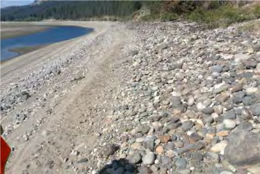
overview facing north
