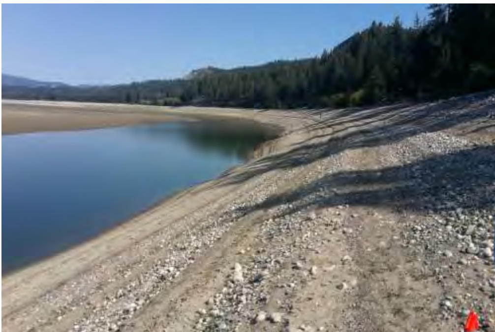
overview facing north
