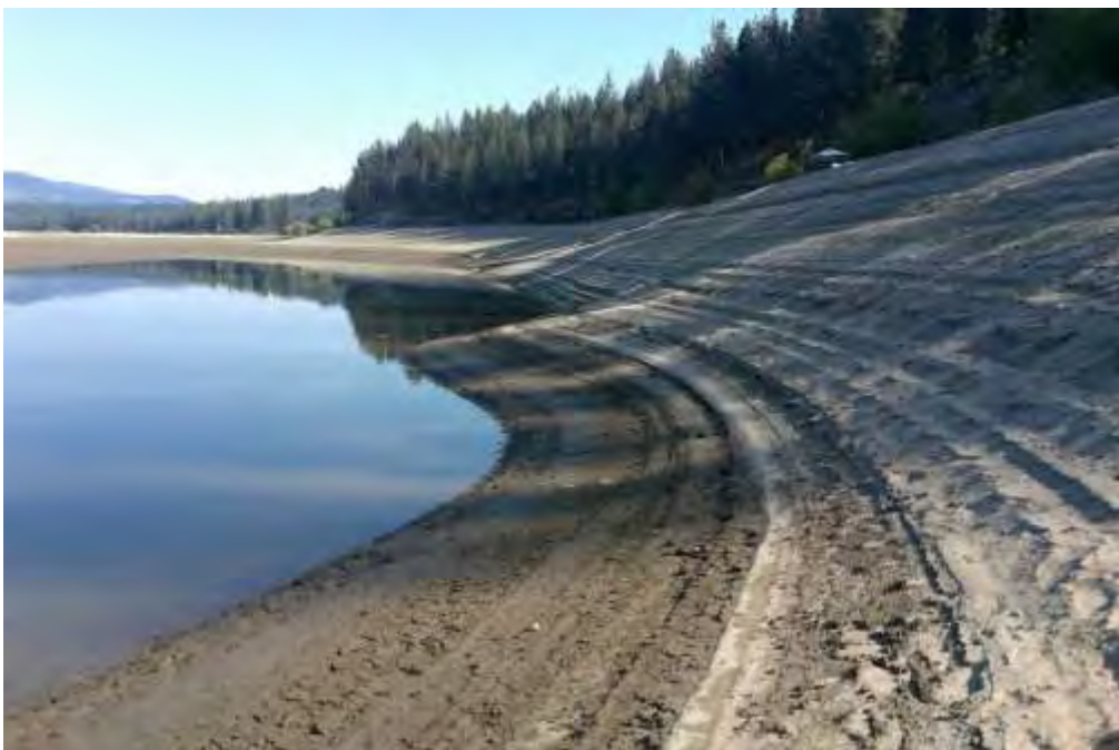
overview facing north
