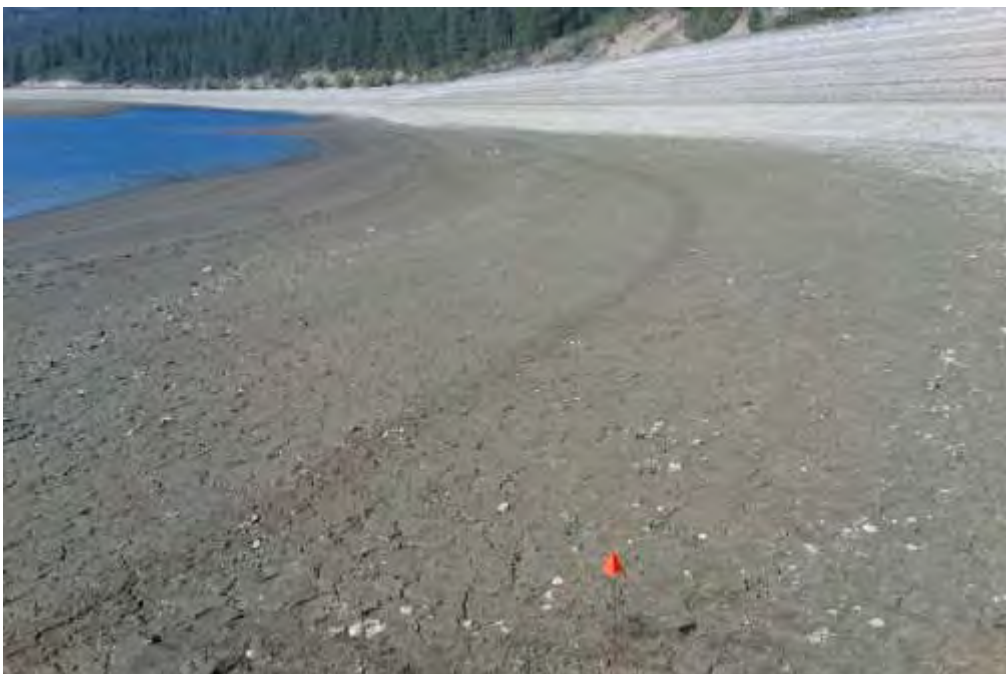
overview facing north
