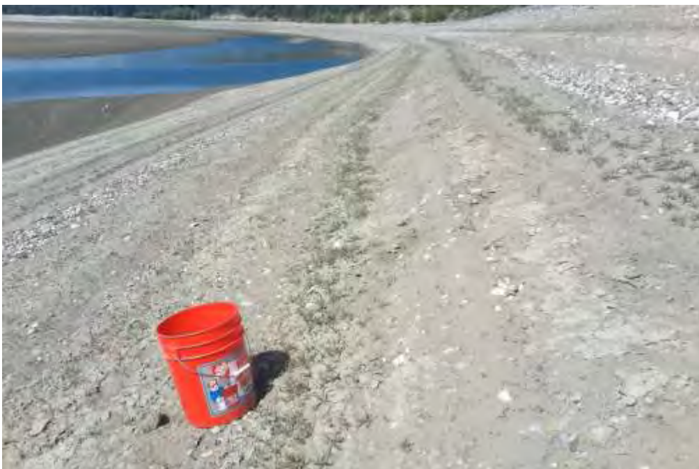
overview facing north
