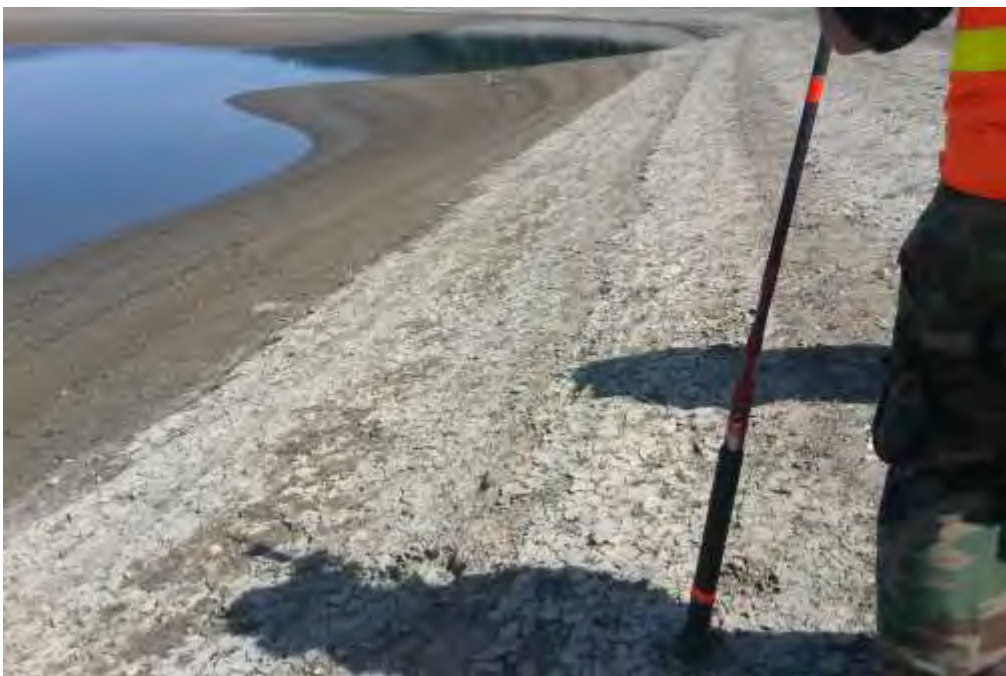
overview facing north
