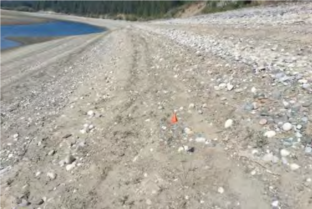
overview facing north
