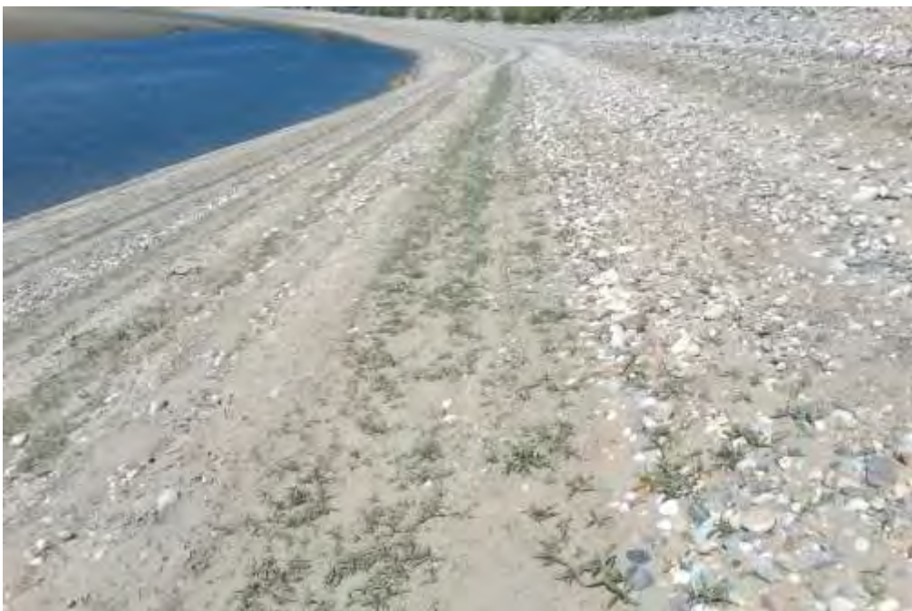
overview facing north
