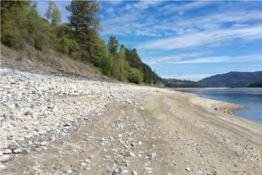
overview facing north
