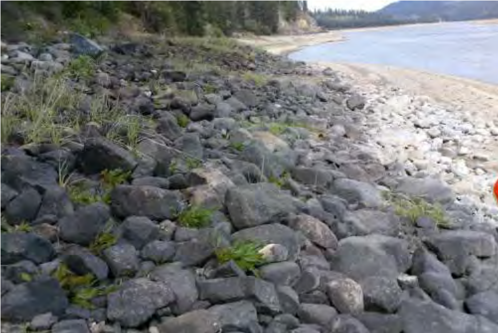
overview facing north
