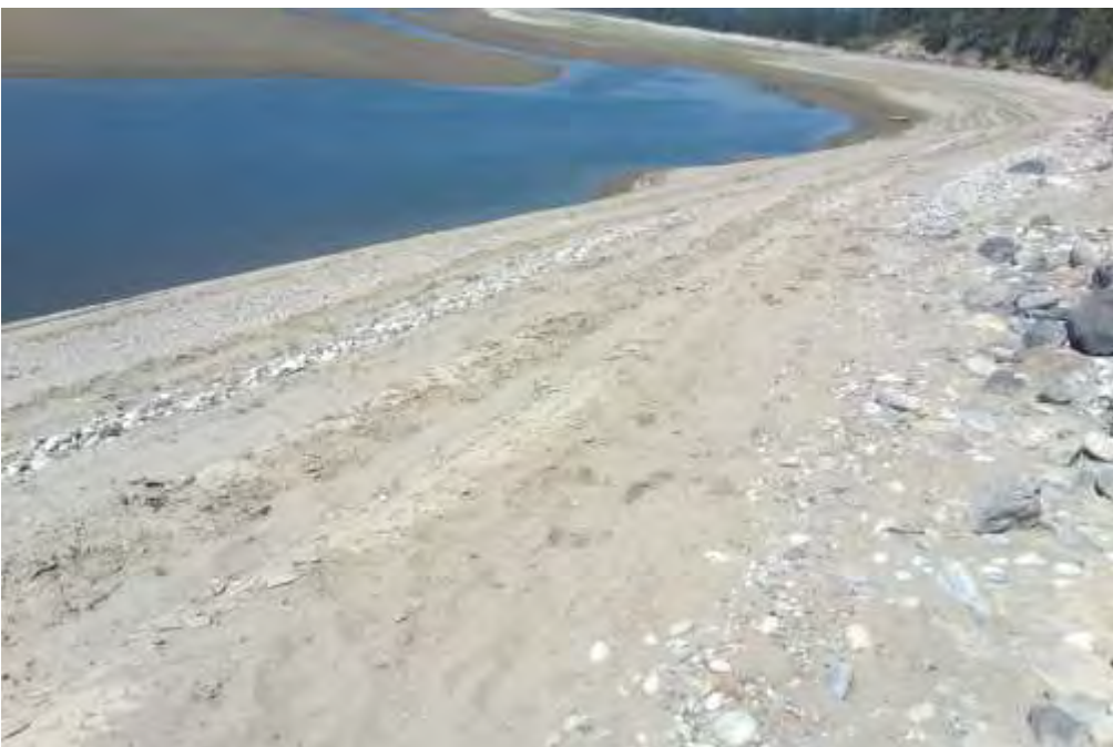
overview facing north
