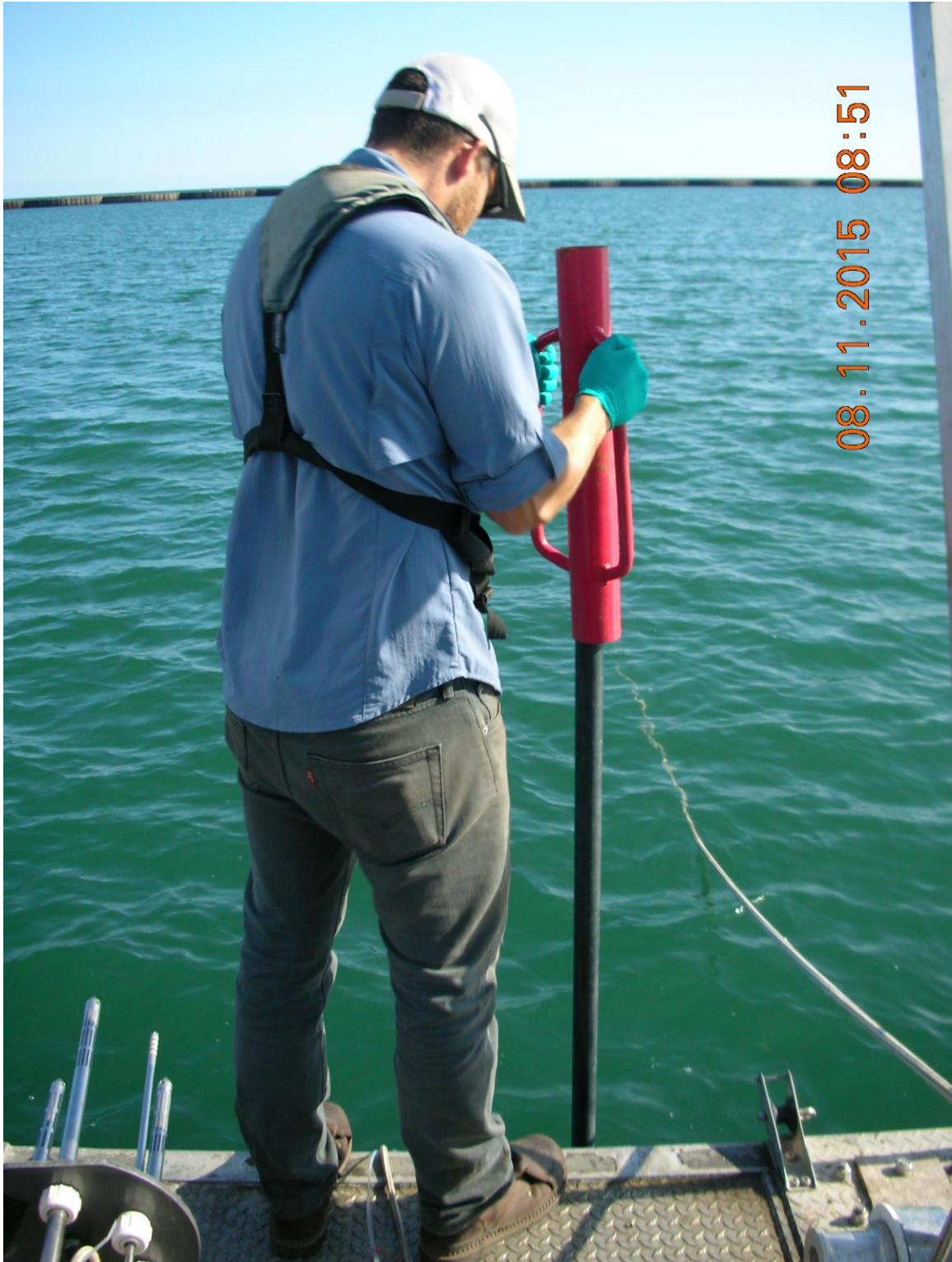
Figure 7. Trident push pole system installation.
