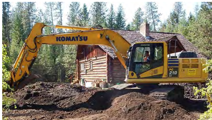
Cleanup activity at residential property
